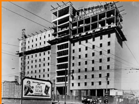
John Vorster Square during construction, 1968 MuseuMAfrica,
